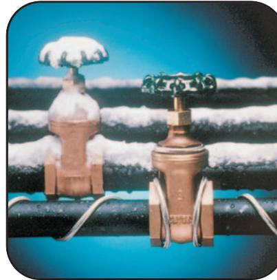
**Constant Wattage Cable** This style of heat trace cable is designed to put out a certain amount of wattage per linear foot at a particular voltage. It is always putting out the designed watts per foot, no matter what the surface or ambient temperature is. This means that in most situations the heating cable is continually pumping heat into the vessel or pipe being maintained or heated. If the heat trace cable is
